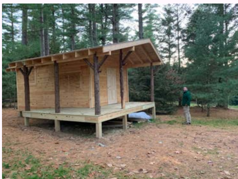
New Whippoorwill Office before application of its "Gucker Green" wardrobe.
